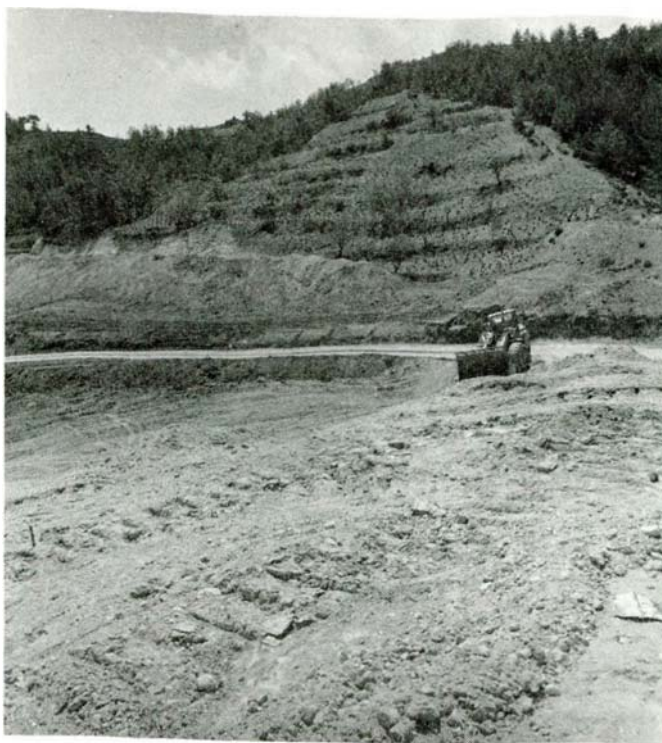
Kyperounda Pond No 2 under construction. WDD Photo D20-11 (23.4.82).
