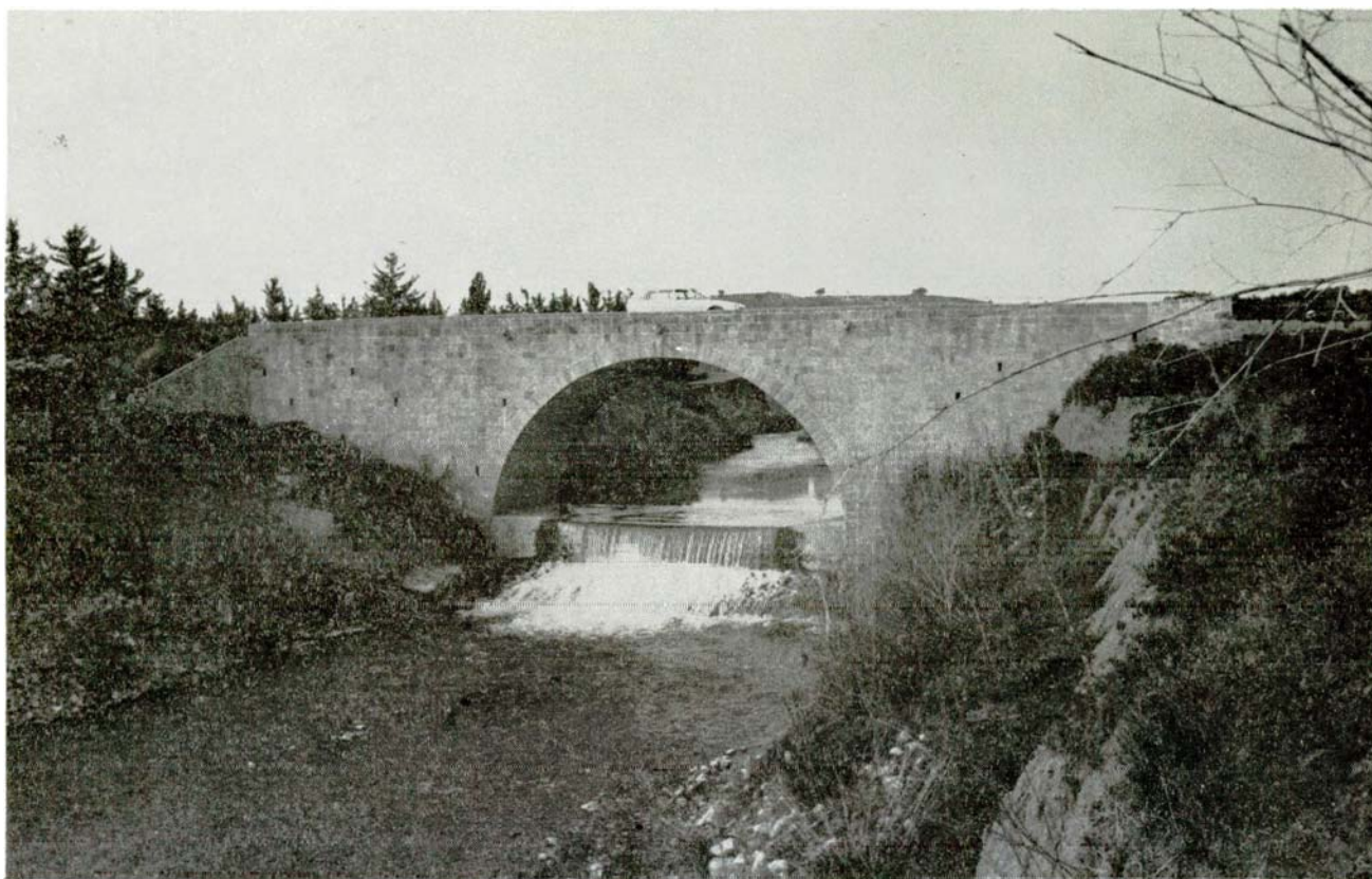
Dhiarizos River gauging station at Kouklia W.D.D. Photo C68EN-29 (18.2.86)
