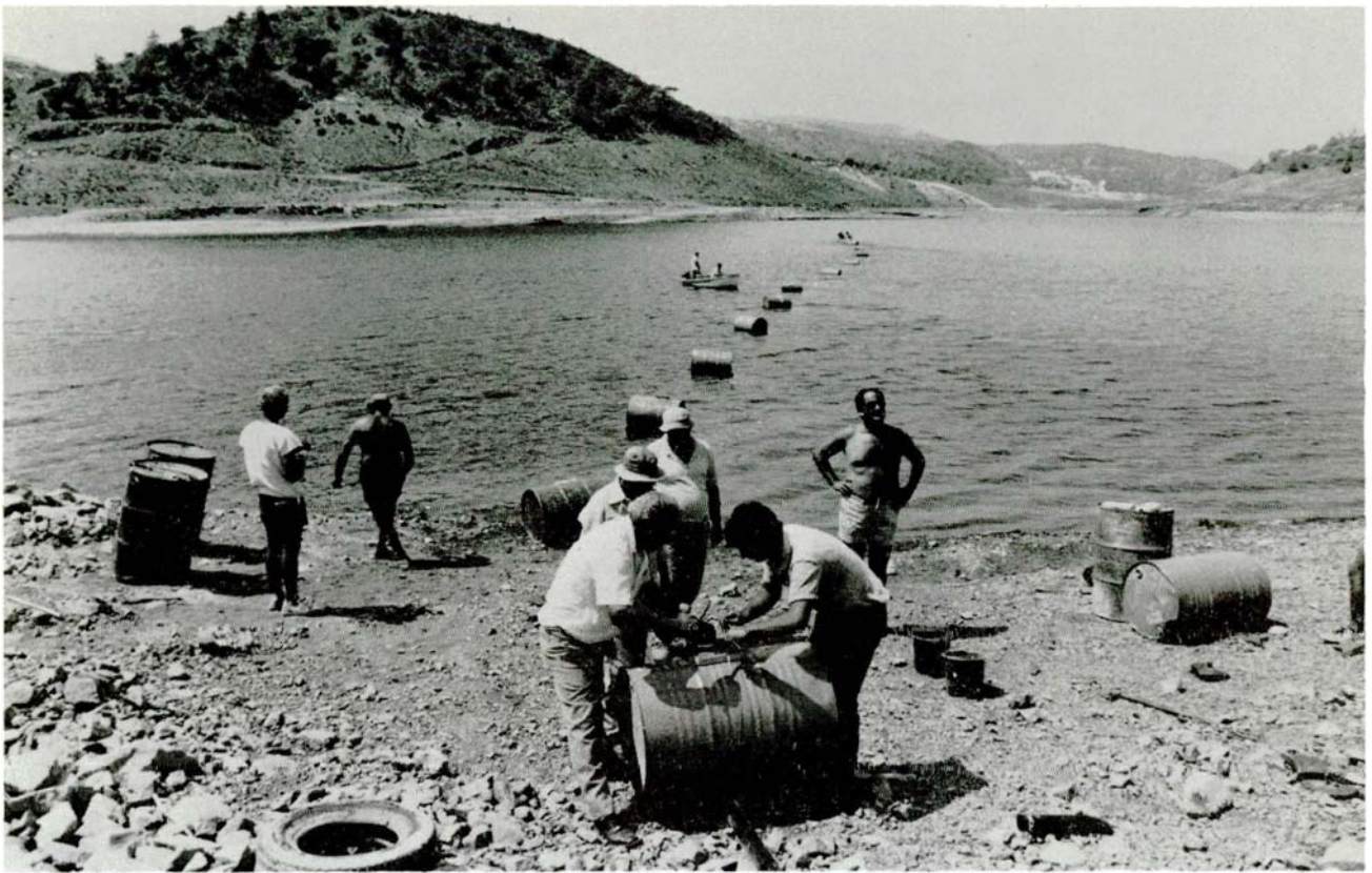
Dhyptomamos Dam aeration operation W.D.D. Photo D10EN-12 (3.9.86)
