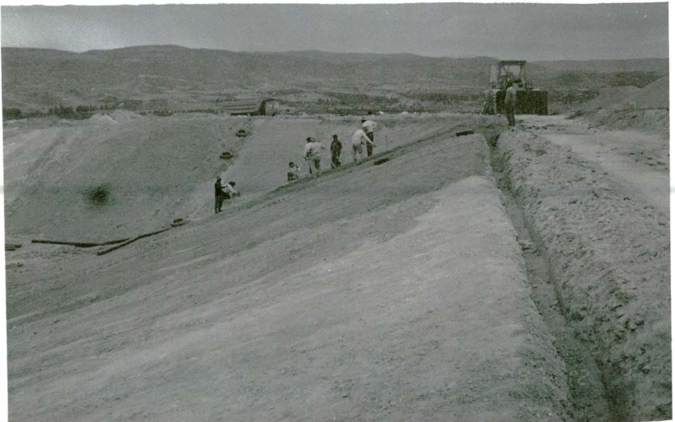
Placing of PVC membrane of Khrysohou West Upper Pond. Contract KC3. (4.12.87).
