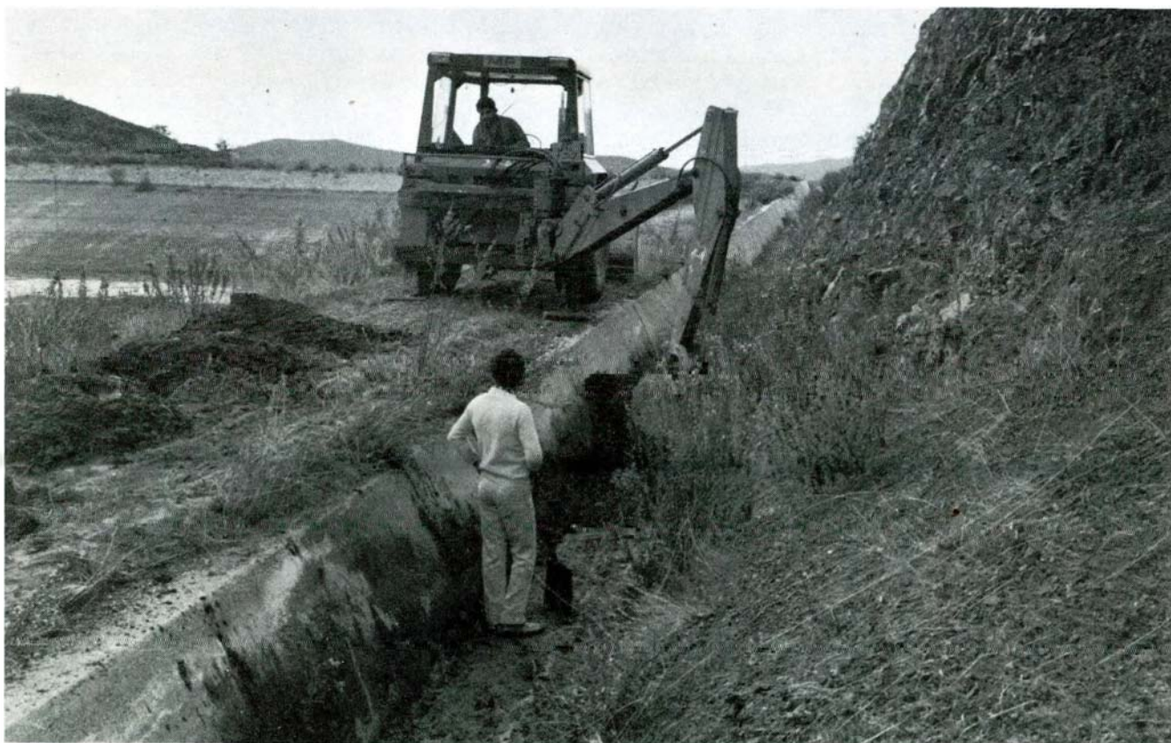
Ora Pond. Cleaning of drainage ditch. (26.11.87).
