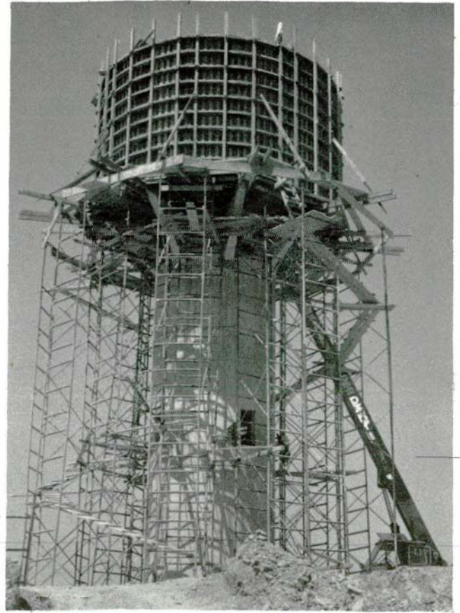
Construction of elevated break pressure tank. Contract KC3 (28.8.87).
