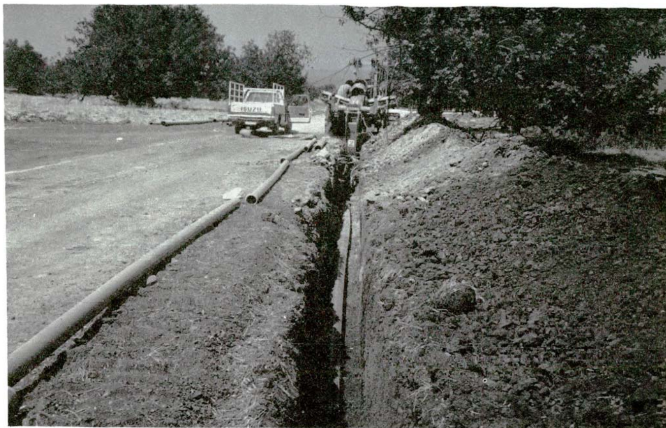
Khrysokhou Irrigation Project. Installation of farm pipelines. Contract KC2 (3.9.87).
