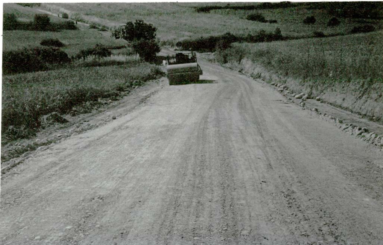
Khrysokhou Irrigation Project. Construction of farm roads. Contract KC2 (21.5.87).
