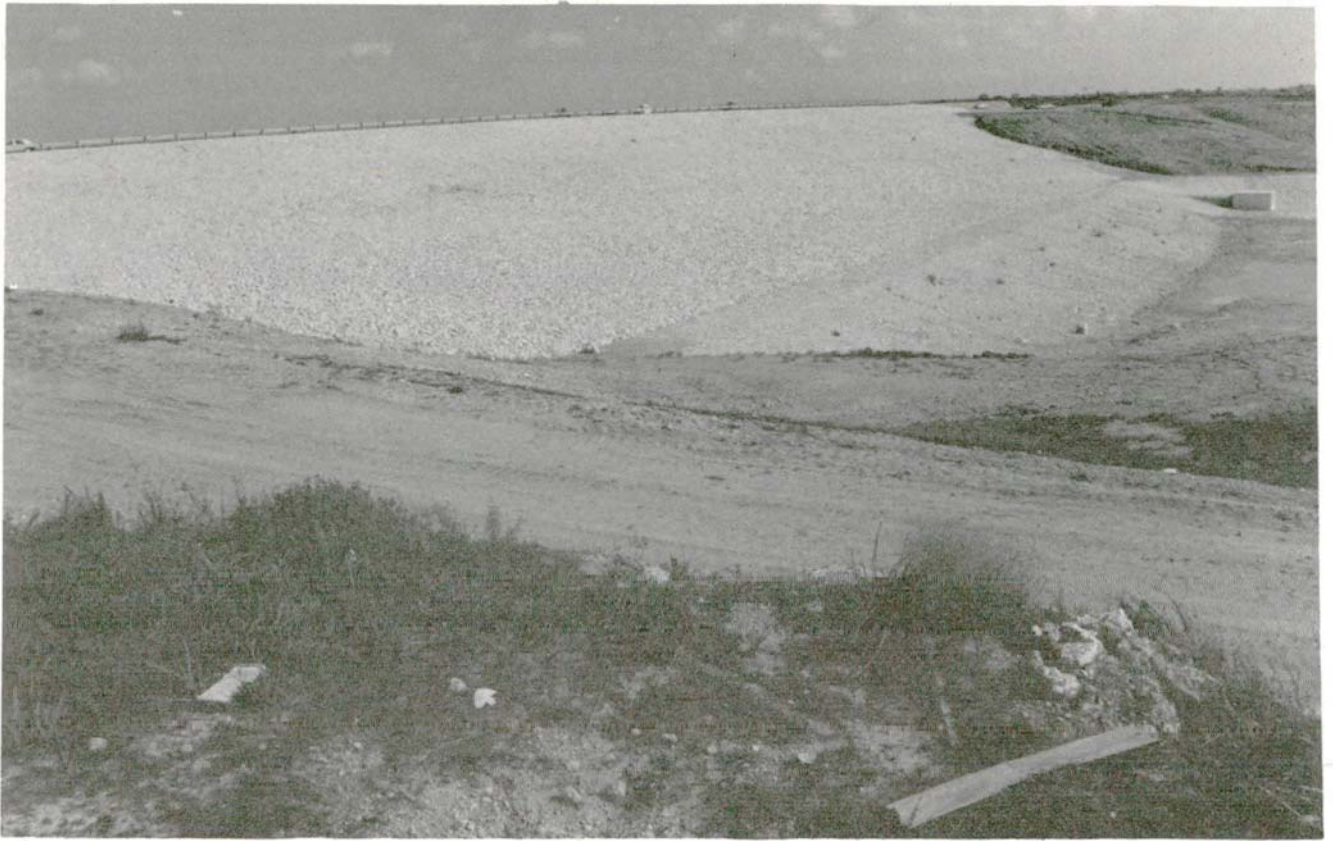
SCP Akhna Dam completed. WDD Photo E58EN-15 (9.2.88)
