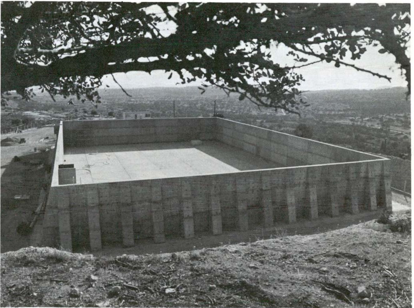
VPP - Balancing reservoir augmenting VPP irrigation requirements with SCP water. WDD Photo D30EN-9 (26.11.86).
