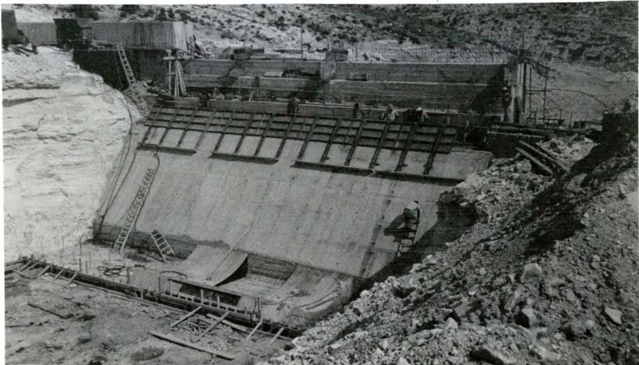
Aradhippou Dam under construction. WDD Photo No. E7EN-16 (17.7.87).
