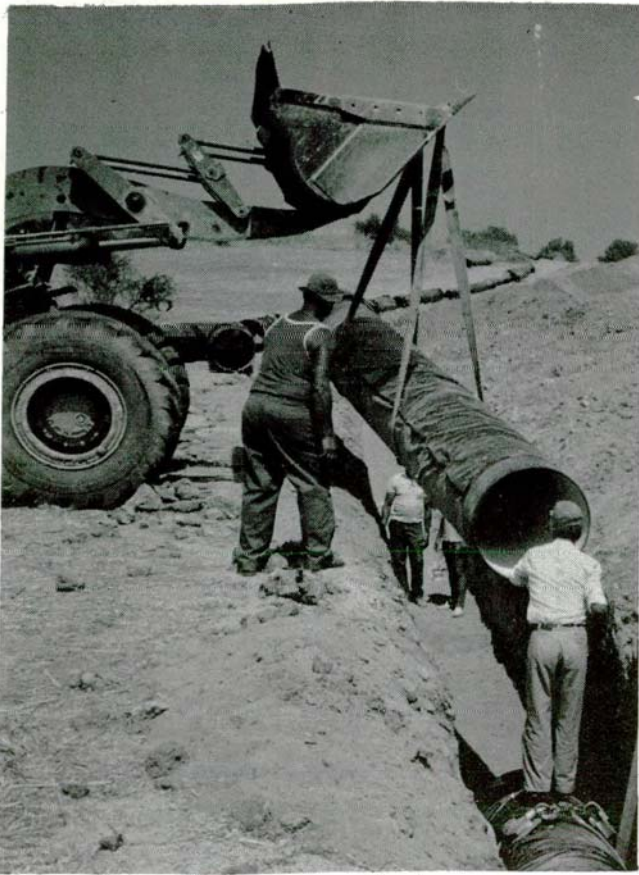
Installation of DI pipes for main conveyor. Contract KC3 (2.9.87).
