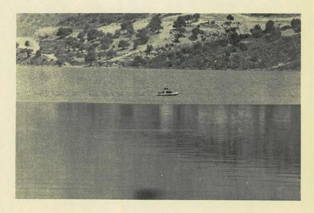
Evaporation Control Experiment — Yermasoyia Dam Application of an Evaporation retardant from a boat. The difference in appearance between the treated and non-treated water surface is very clearly illustrated.
