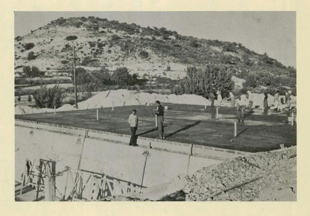
Casting of Roof Slab on 450,000 gallons capacity underground Reservoir at Khirokitia for Famagusta Water Supply.
