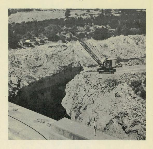
View of extensive silting of reservoir. Broken metal structures were fished out by crane.
