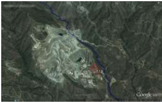
ΕΕΑ Λ1β - SKYRAMONT QUARRIES LTD
