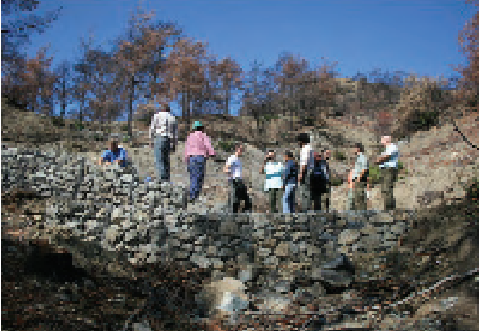
Construction of retaining walls on a practical session
