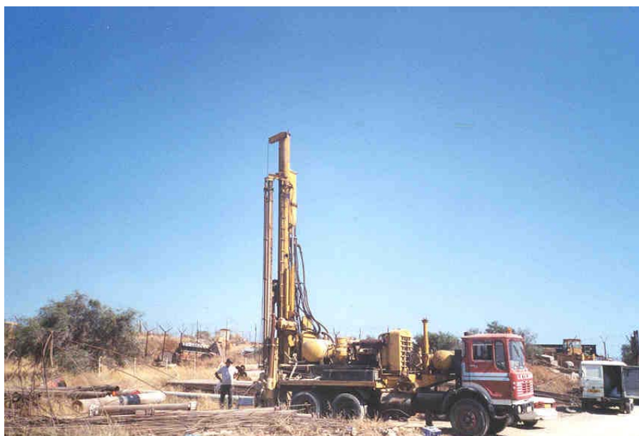
Figure 4.1. Drilling at the Askarel site in June 2001.
