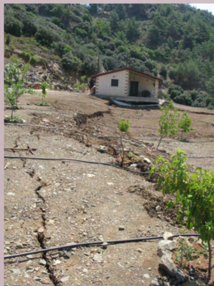
5. Instability on artificial slope at Ayious Vavatsinias village
