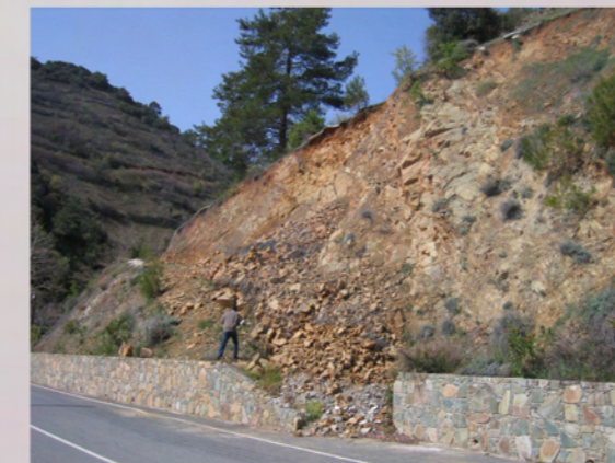
4. Landslide occurring on rock mass of diabase sheeted dykes at Yerakies village
