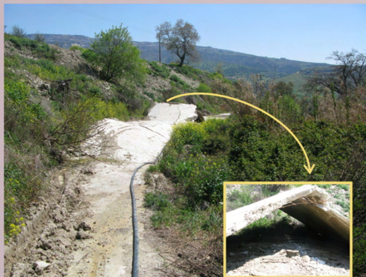
6. Rural road at Kritou Marottou village which was affected from the adjacent landslide. The additional picture down on the corner shows in detail the toe of the landslide
