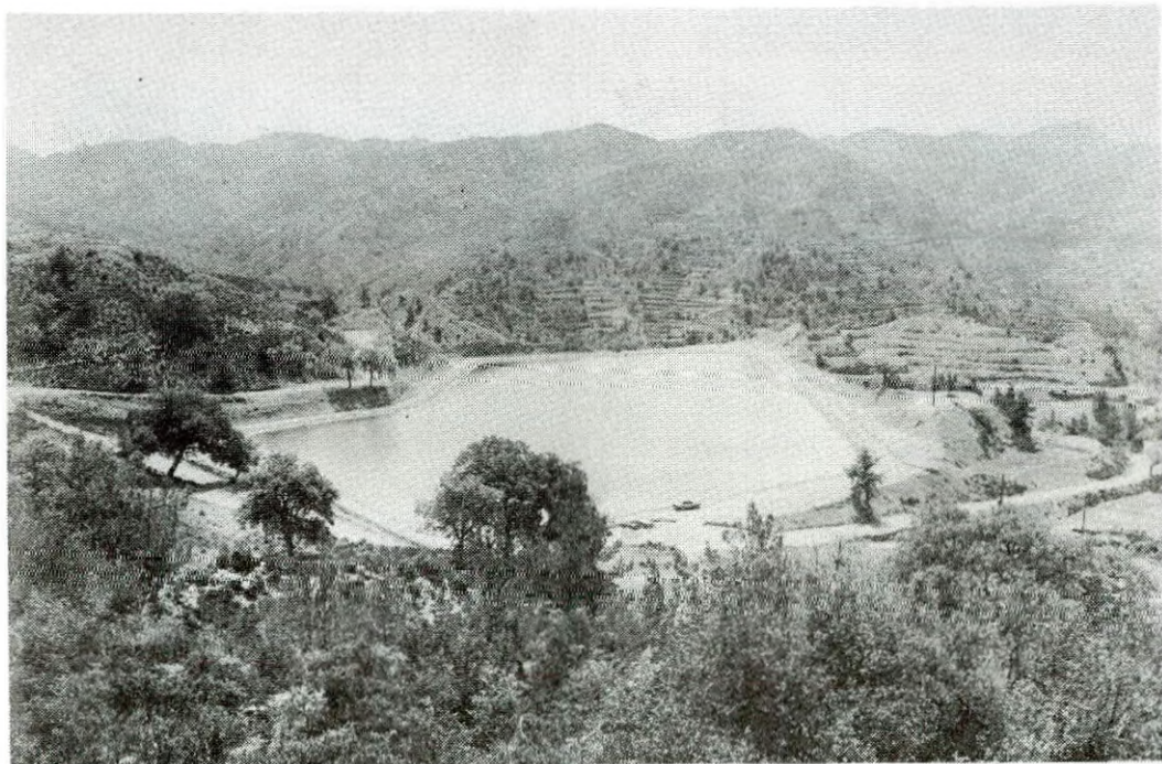
The first filling of Kato Mylos Pond was during December 81 to January 82. Water is diverted to the pond from a stream through a 150 mm dia, 2 km long gravity pipeline. Water from the borehole is used to irrigate the higher lying areas of the Vatera Irrigation Division with the possibility of feeding also the pond which commands the low lying areas of the Division. WDD Photo D20-8 (23.4.82)
