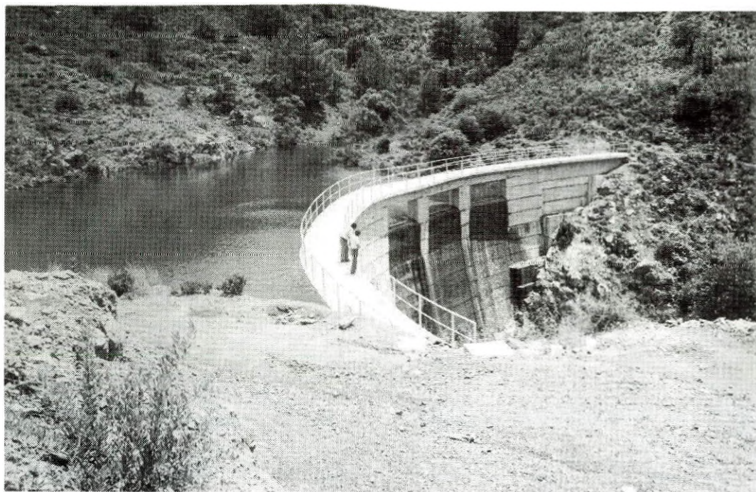
Ayii Vavatsinias is a small arch dam of 54,000 m 3 capacity. With Ayii Vavatsinias Pond also completed in 1981 they will irrigate an area of 180 donums of land to be planted mainly with citrus and vegetables. The first impoundment of both structures belonging to Pitsilia Integrated Rural Development Project was in March 1981. WDD Photo D24-6 (3.6.82)
