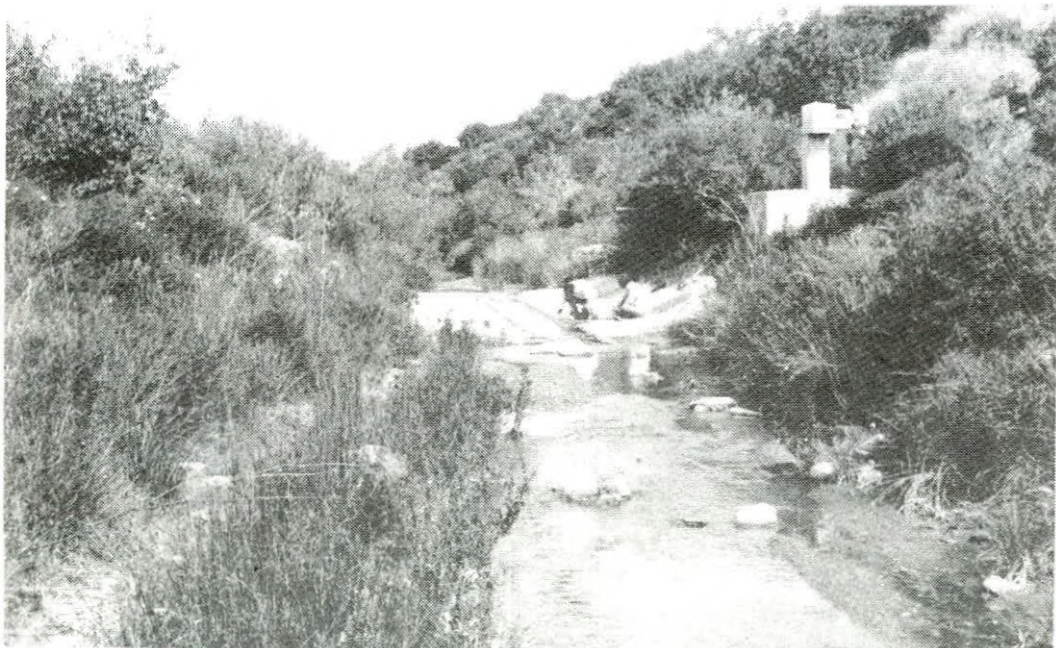
Flow gauging station on Syrkatis stream at the inflow of Dhypotamos Dam. This dam will be built on the confluence of Syrkatis and Mylous tributaries of Pendaskinos River. WDD Photo 97EN-19.
