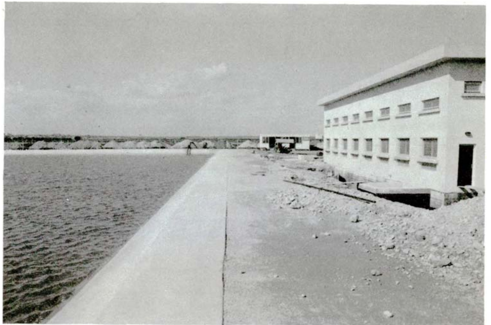
SCP Contract C6. Reservoir and pumping station of CDP VII. WDD photo F50EN-4A. Taken on 3.11.88.
