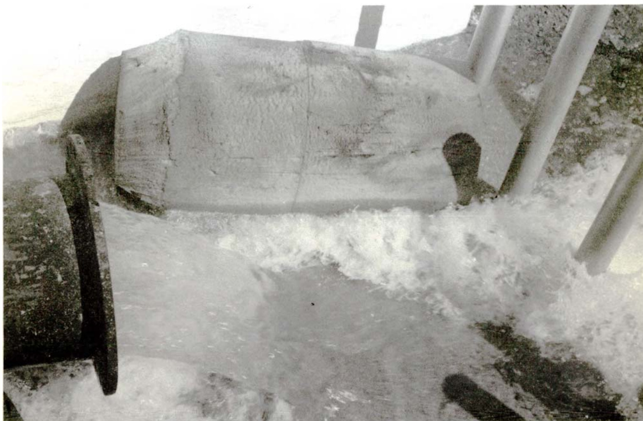
Swabbing of the Khirokitia-Phrenaros pipeline.
