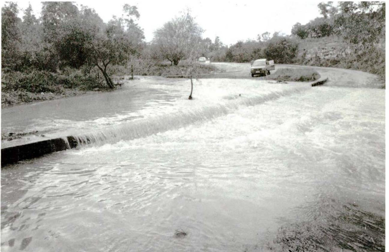
Floods at the Pedhieos Irish bridge in Nicosia just below the Presidential Palace. WDD photo E72EN-23. Taken on 8.3.88.
