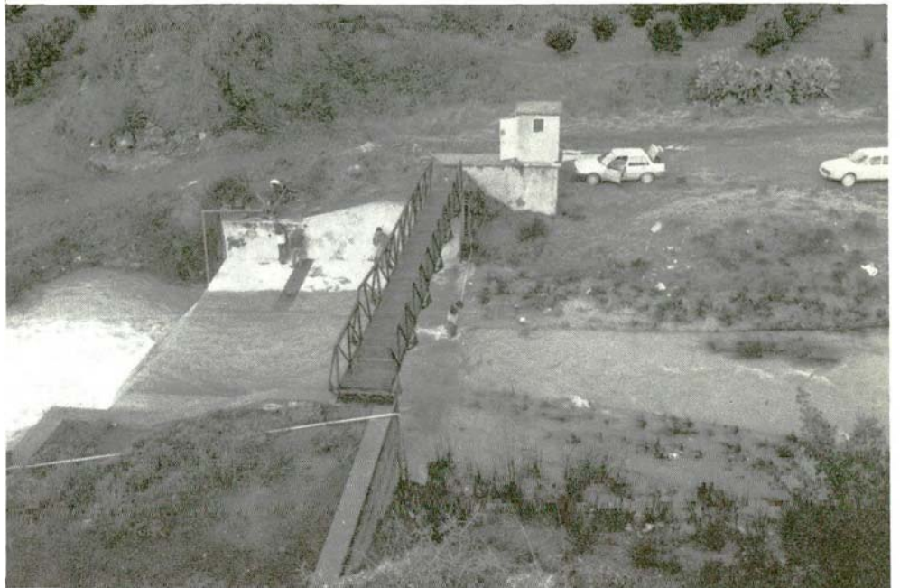
Ezousas river flow gauging station near Kannaviou. WDD photo E52EN-23. Taken on 26.1.88
