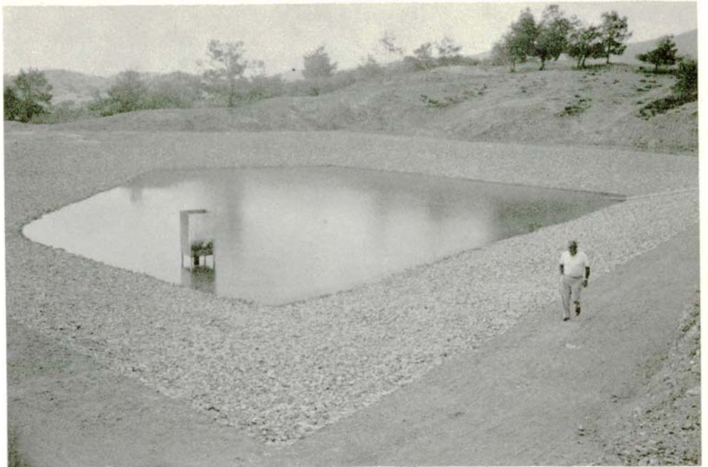
Kakopetria sewage effluent storage pond. WDD photo F51EN-1. Taken on 27.10.88.
