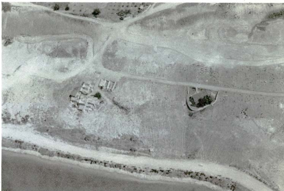
What remained of Khalassa old village after construction of Kouris dam. All the houses were demolished as the village is to be inundated by the dam reservoir. In addition the underlying soil was used as fill for the 9.4 MCM dam embankment. It was agreed though, not to demolish the old church and grave yard which will be partly flooded. WDD photo F35EN-2. Taken from the air on 30.8.88.
