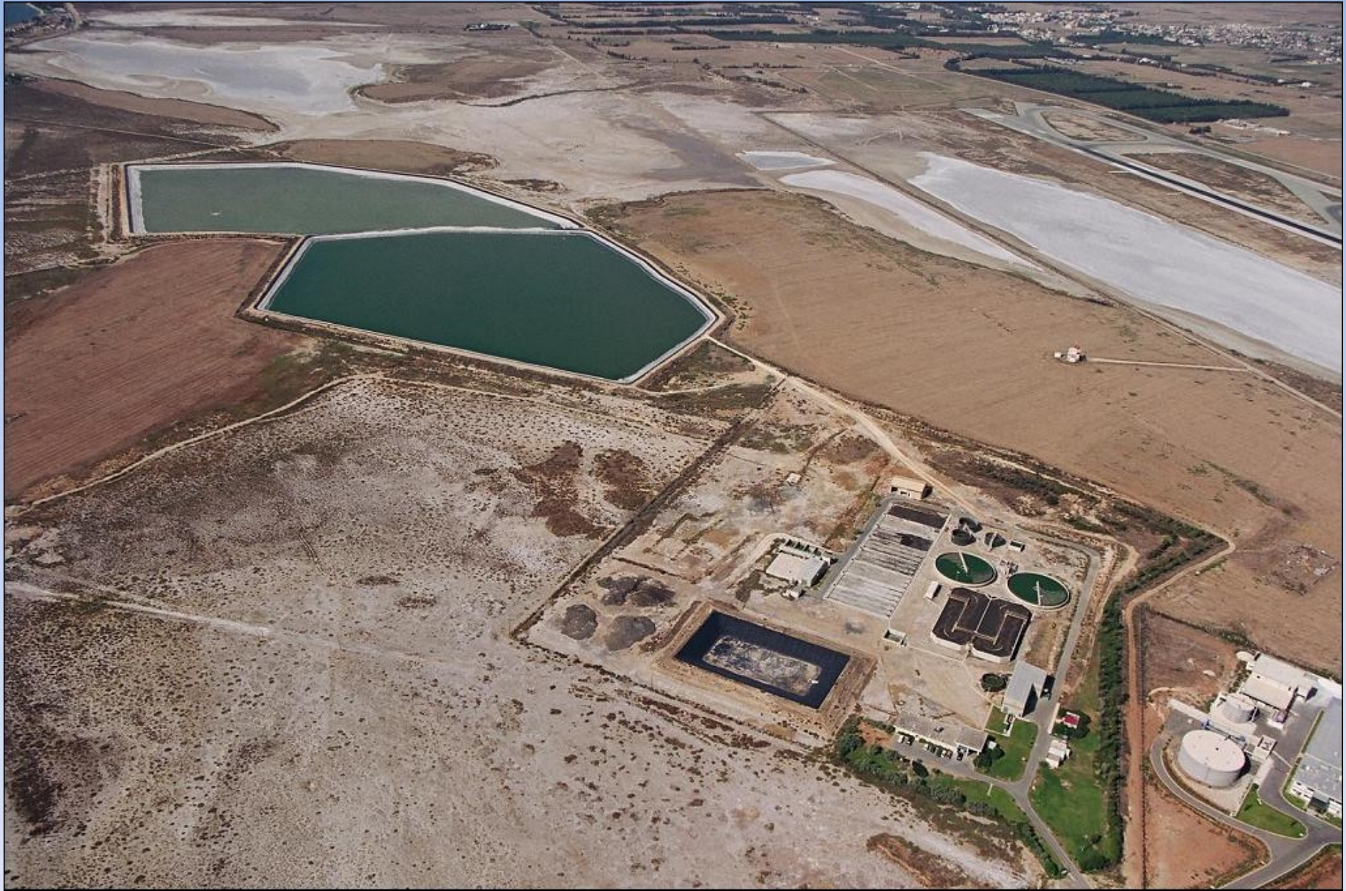
LARNACA WASTEWATER TREATMENT PLANT-SBL
