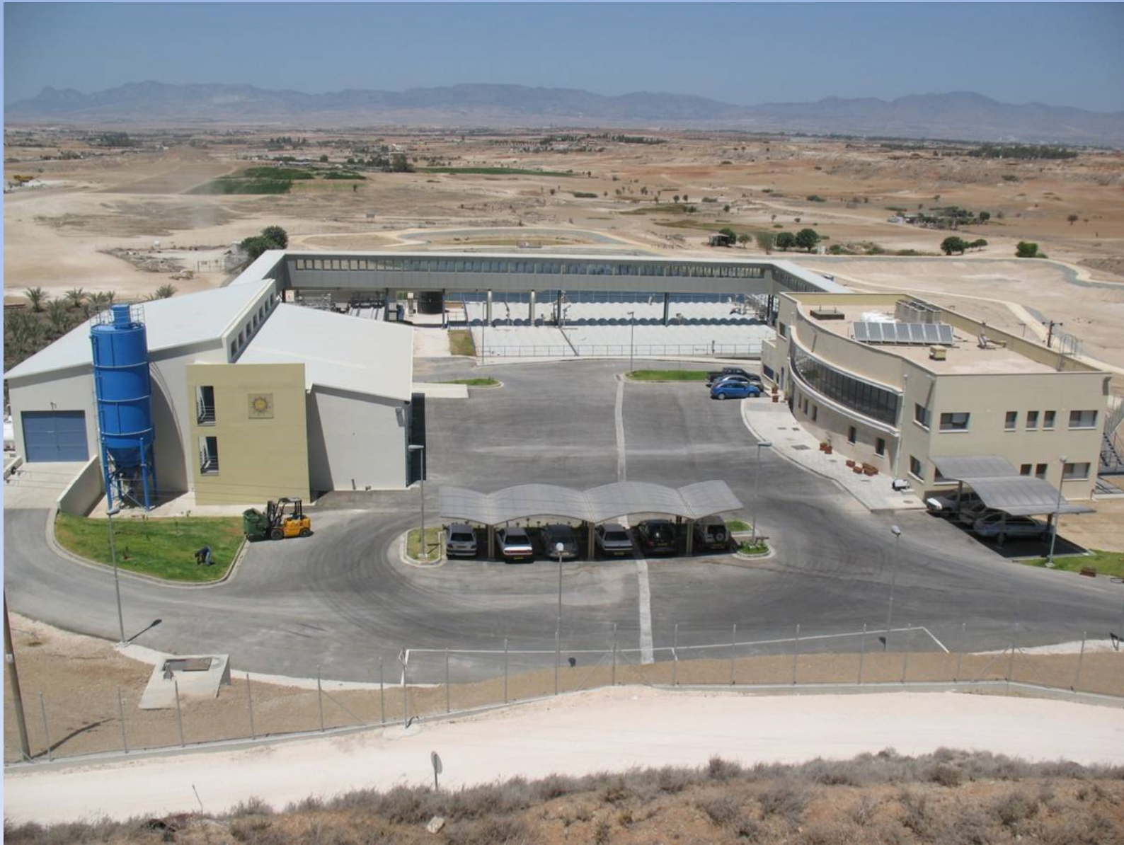
ANTHOUPOLIS WASTEWATER TREATMENT PLANT -SBN
