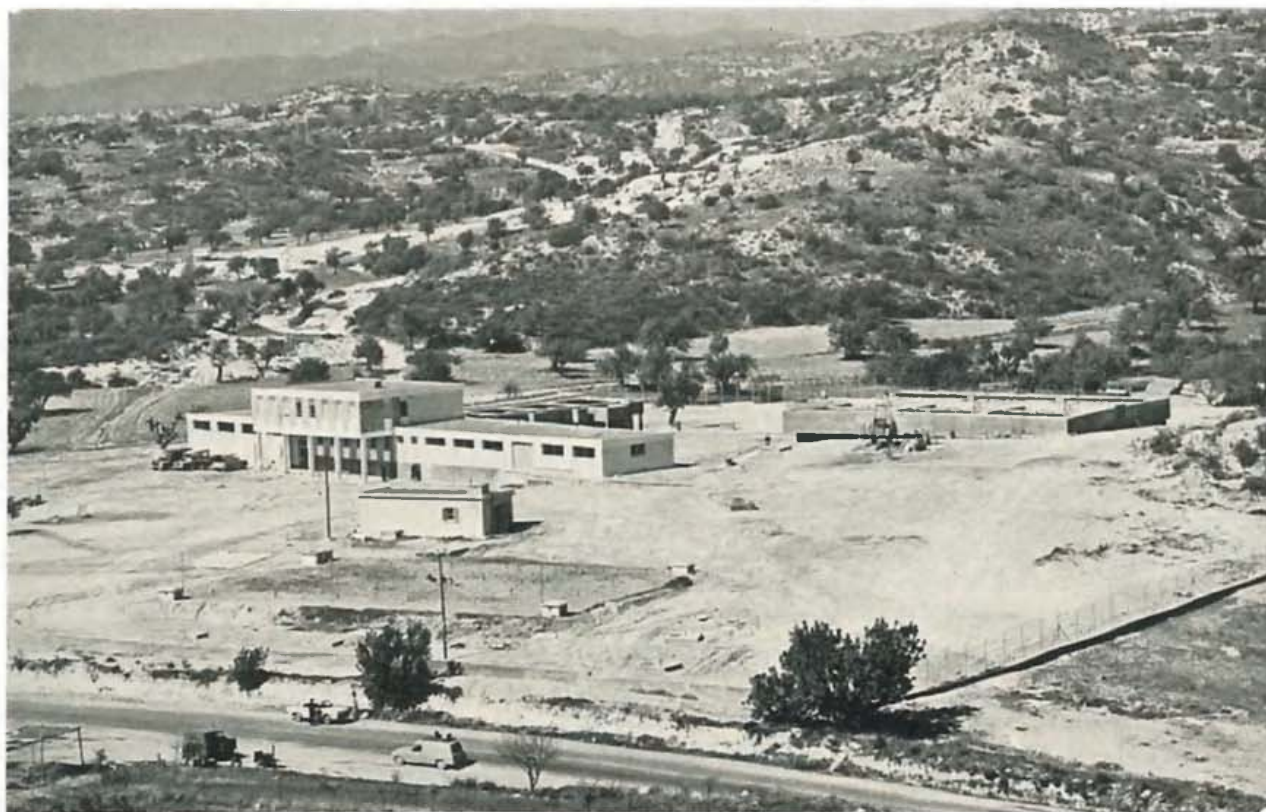
Khirokitia water treatment plant.
