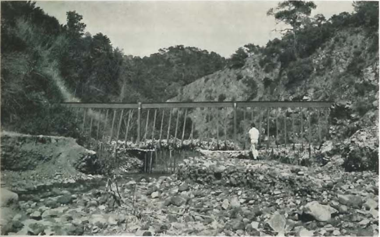
Trimiklini dam. — Upstream silt trap.
