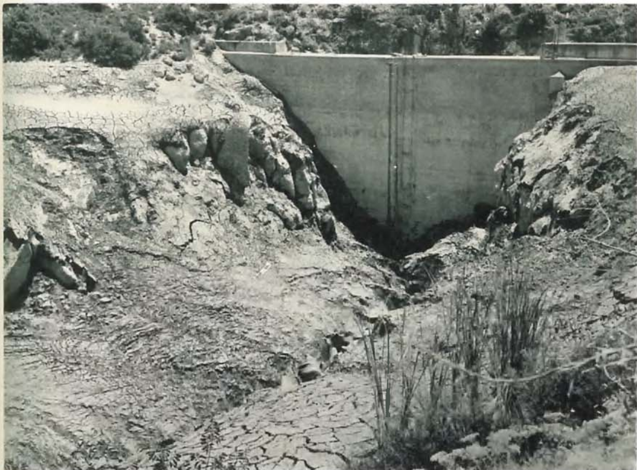
Trimiklini dam in May 1969 showing silt deposited in the reservoir from erosion of the Asbestos Mines dumps upstream. The depth of the silt at the lowest point is 8 m.
