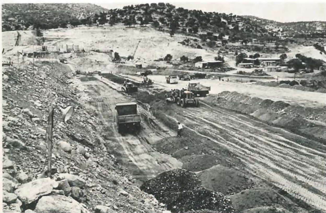
Yermasoyia dam under construction.
