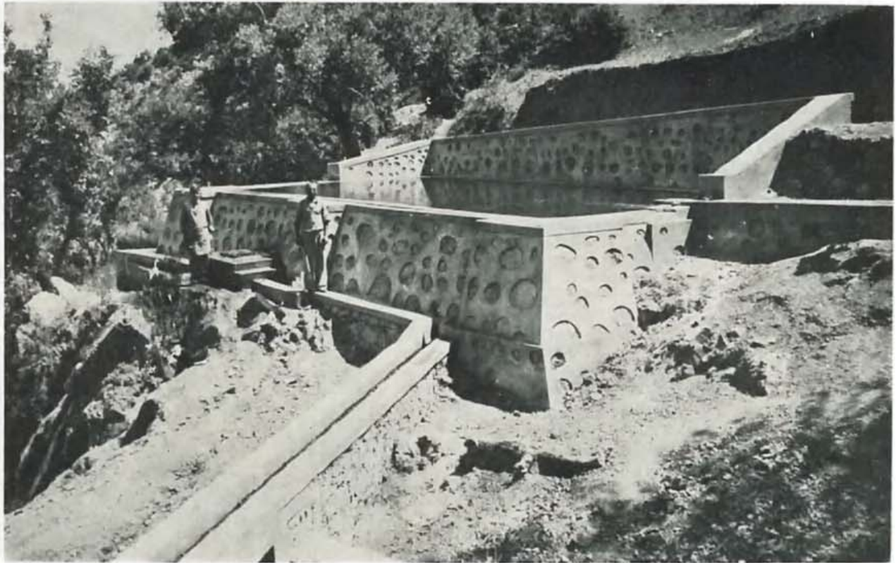
Masonry reservoir and intake channel
