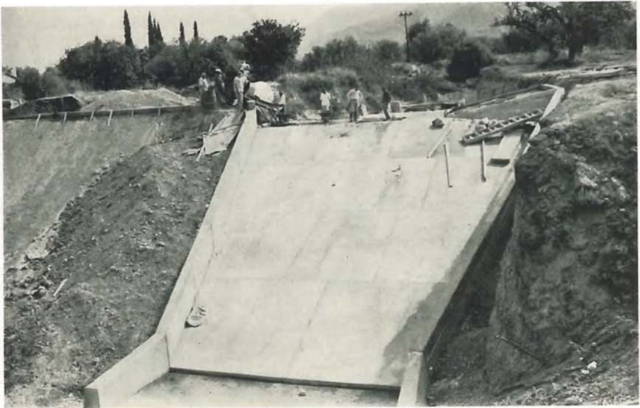
Recharge dam at Karakoumi.
