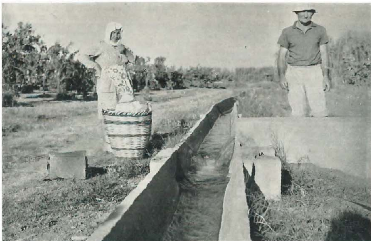
Precast concrete polycentric irrigation channels at Morphou.
