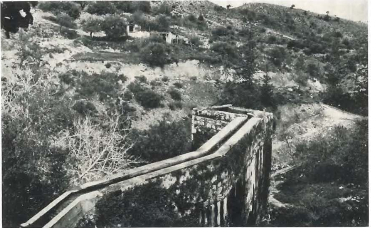
Flour Mill using hydropower for the operation of grinding wheel.
