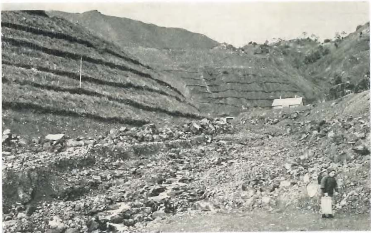
Old waste dumps at Amiandos Mines showing timber staking and tree planting for the prevention of erosion
