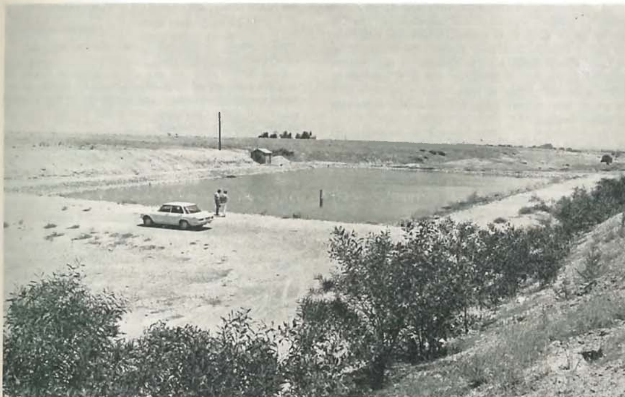
Margo Reservoir: Excavated and earth fill. Polythene sheet cover 0.25 mm thick. Capacity 60,000 m 3 .
