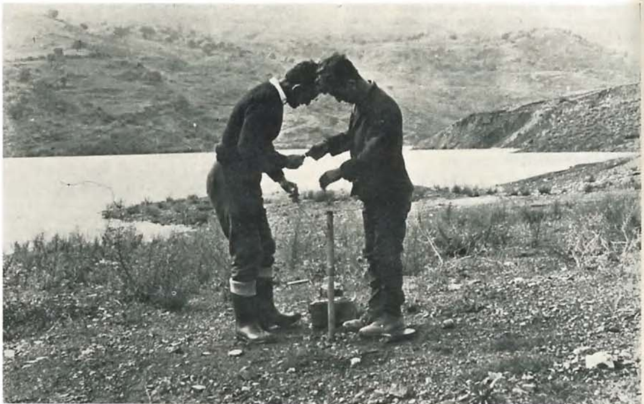
Piezometric observations on the right abutment.
