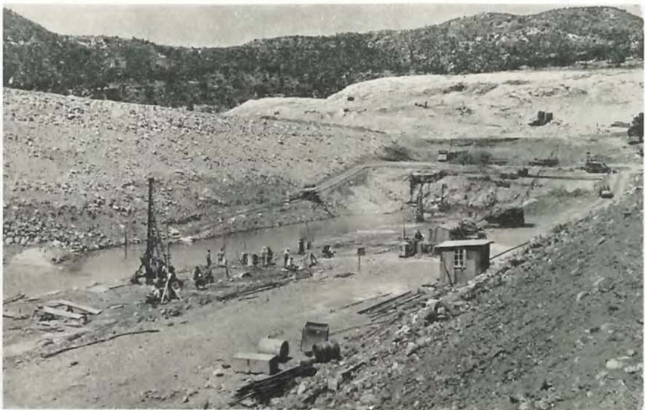
Cut-off trench excavation with alluvial grouting.
