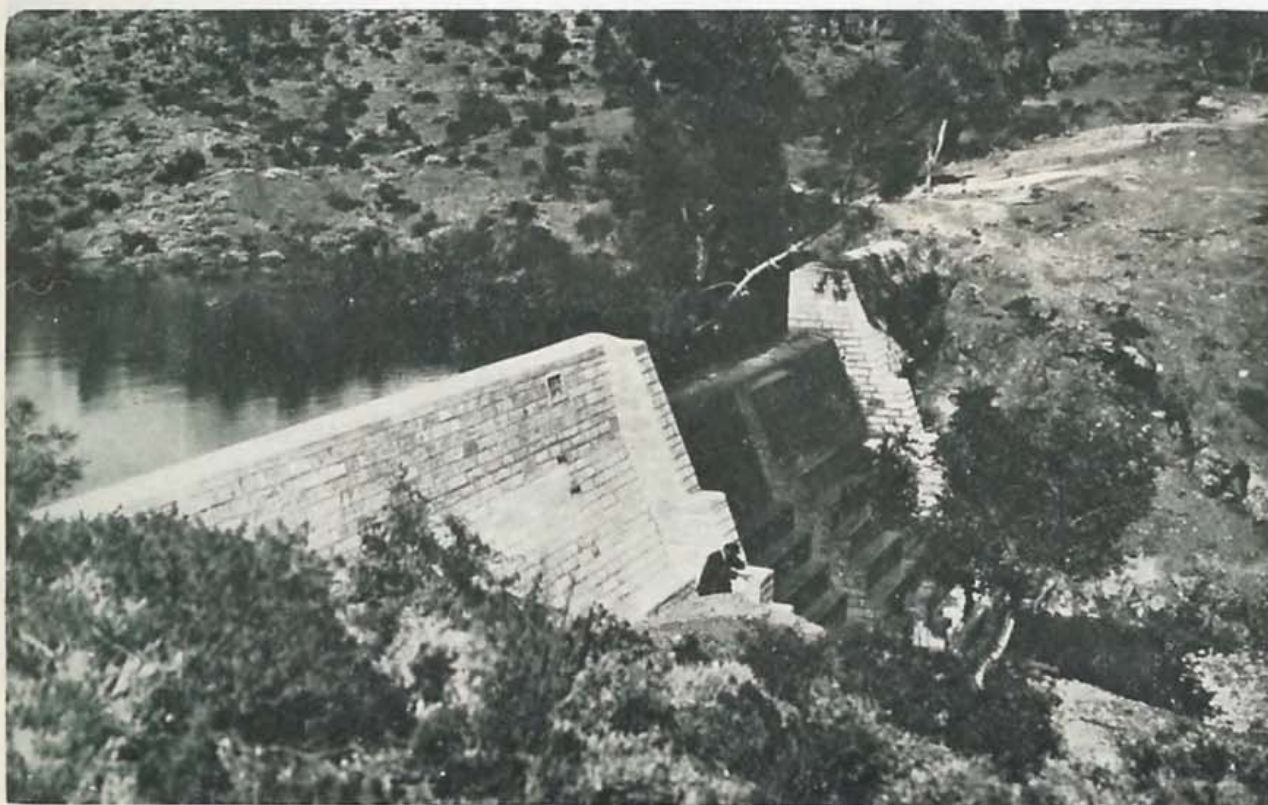
The Kophinou masonry dam.
