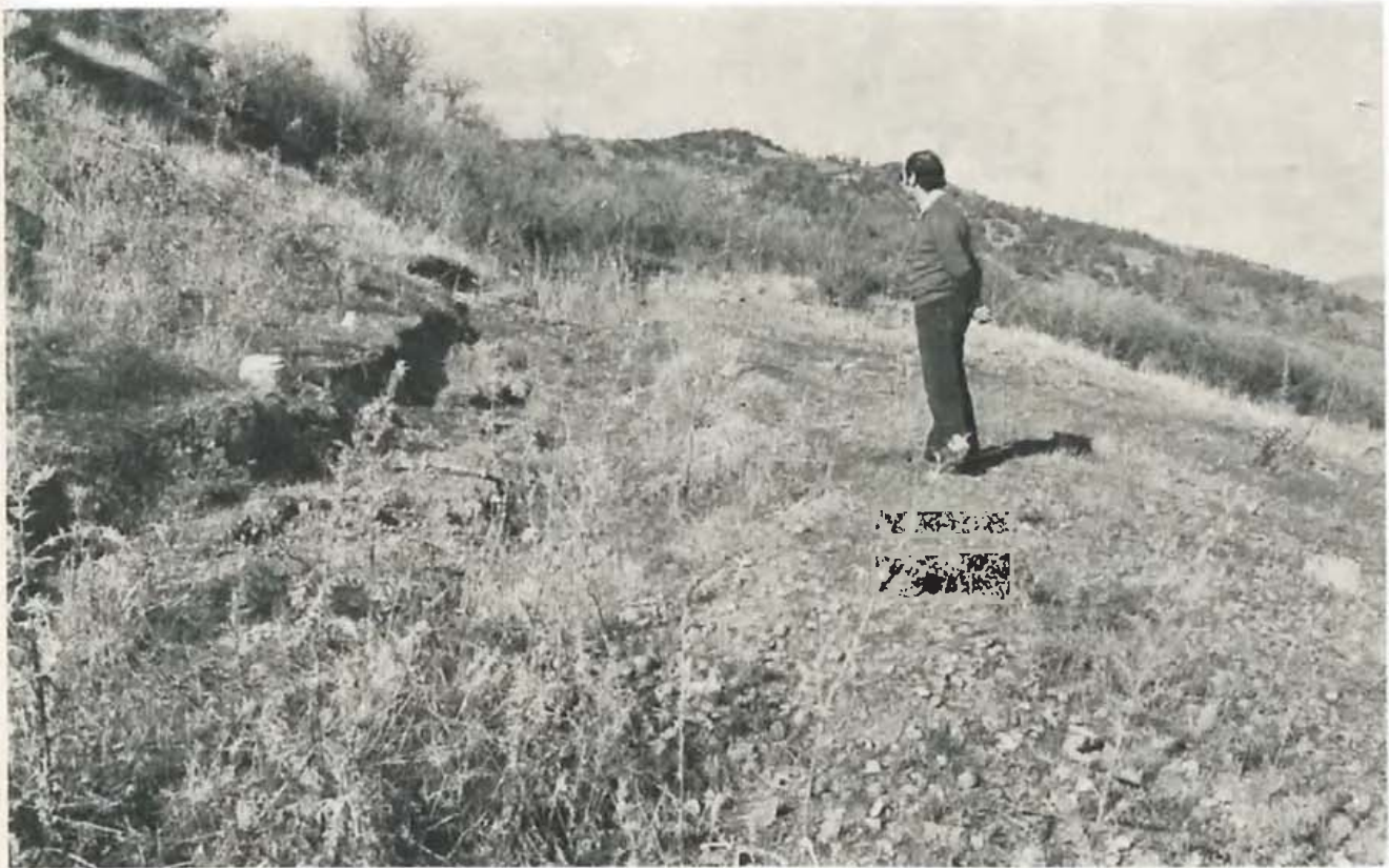
Crack on the overburden overlying the diabase of the Western flank.
