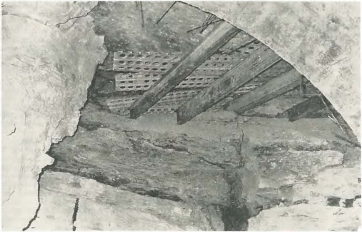
Excavation of tunnel showing solution channels in the sandstone.
