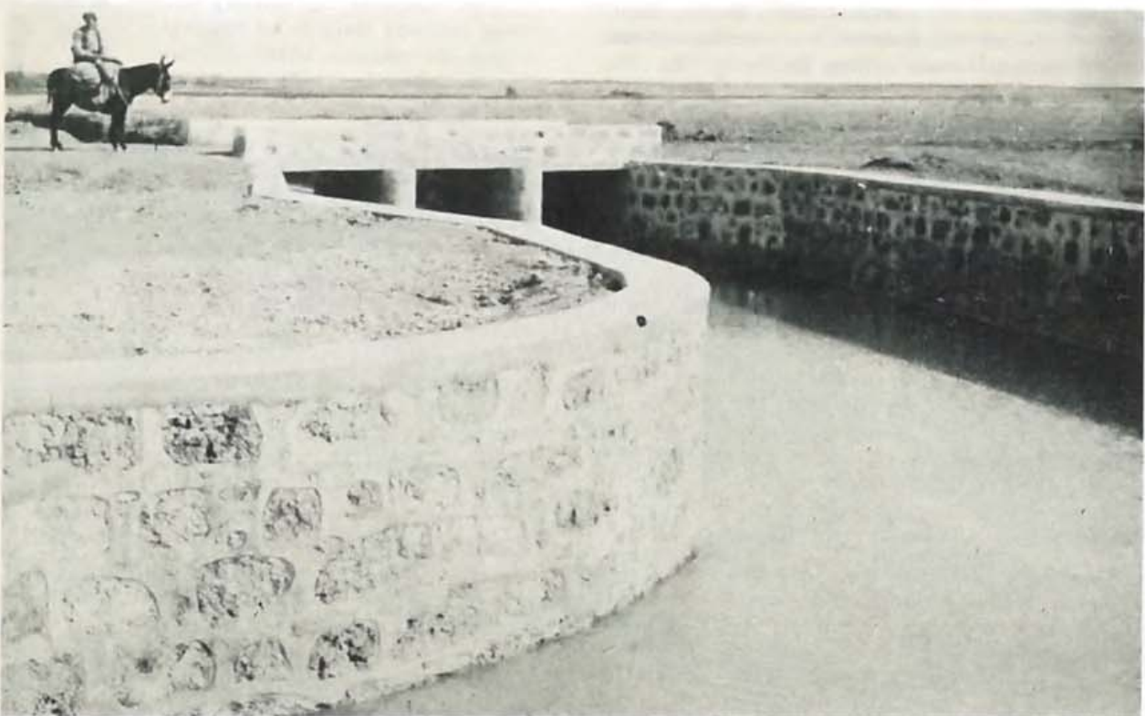
Masonry conveyor channel and bridge.
