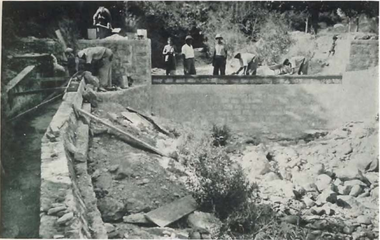
Masonry river diversion weir and intake channel.
