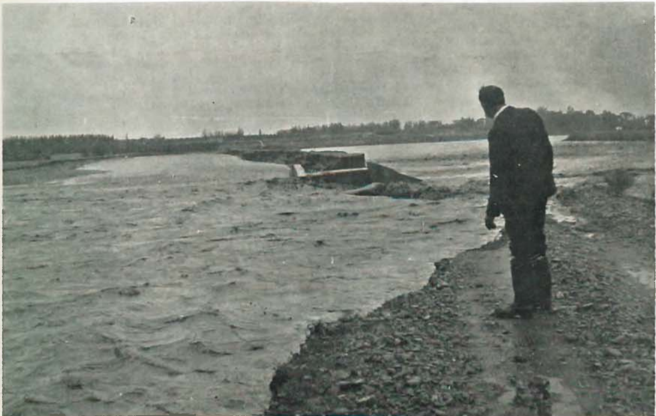
Overflowing spreading grounds on the left with flooded river course on the right.
