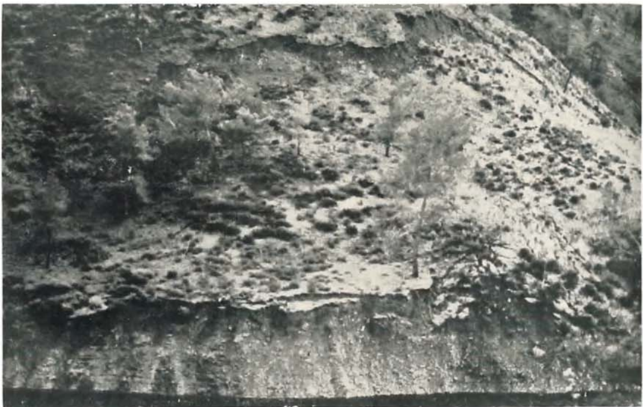
Pomos dam reservoir. — Upstream slide area.
