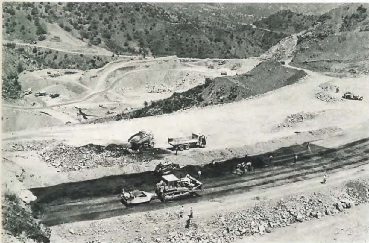
Lefkara rockfill dam under construction.
