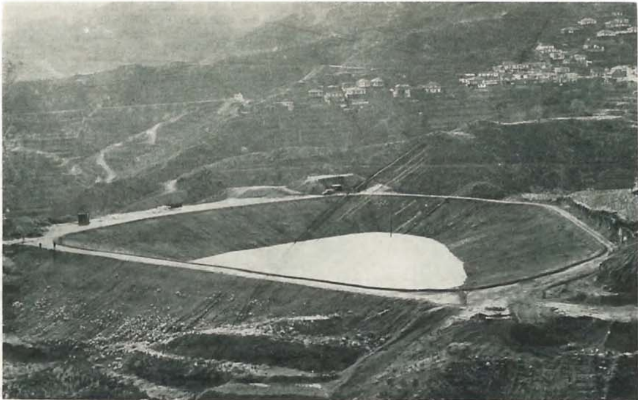
Kyperounda Reservoir 1400 m asl. Excavated and earth fill. Polythene sheet cover 0.25 mm thick. Capacity 5,000 m^3 .
