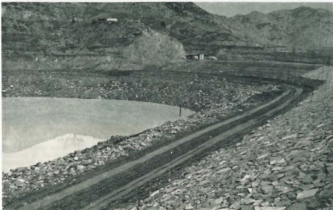
Clay blanket on original rip-rap.
