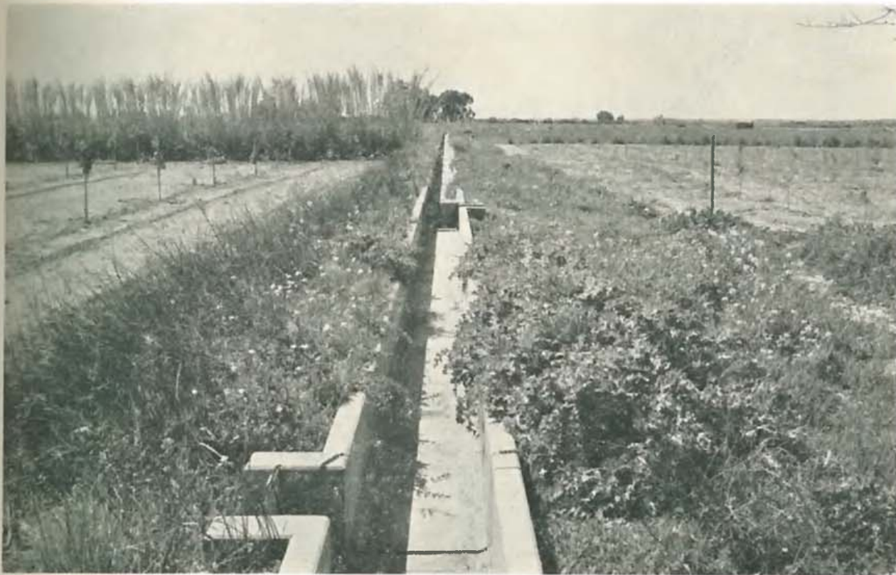
Rectangular R.C. irrigation channel.
