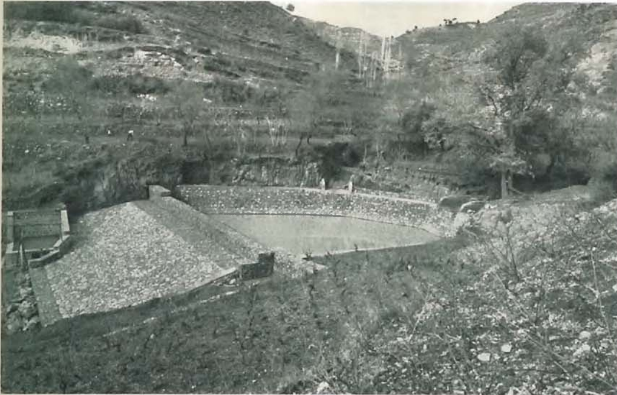
Silt trap upstream of Agros dam.
