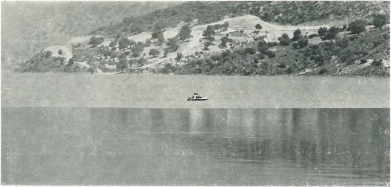
Application by boat of Cetyl Alcohol in the Yermasoyia Dam Reservoir for the reduction of evaporation rate. In the foreground the treated part can be seen with the film cover showing distinctly.
