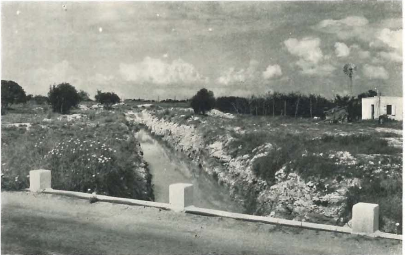
The Paralimni lake recharge conveyer canal.
