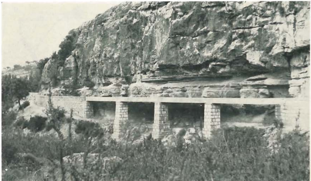
The Kandou masonry - concrete irrigation aqueduct.
