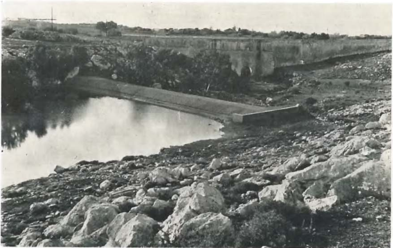
Ayia Napa typical recharge dam. An old aqueduct can be seen in the background.
