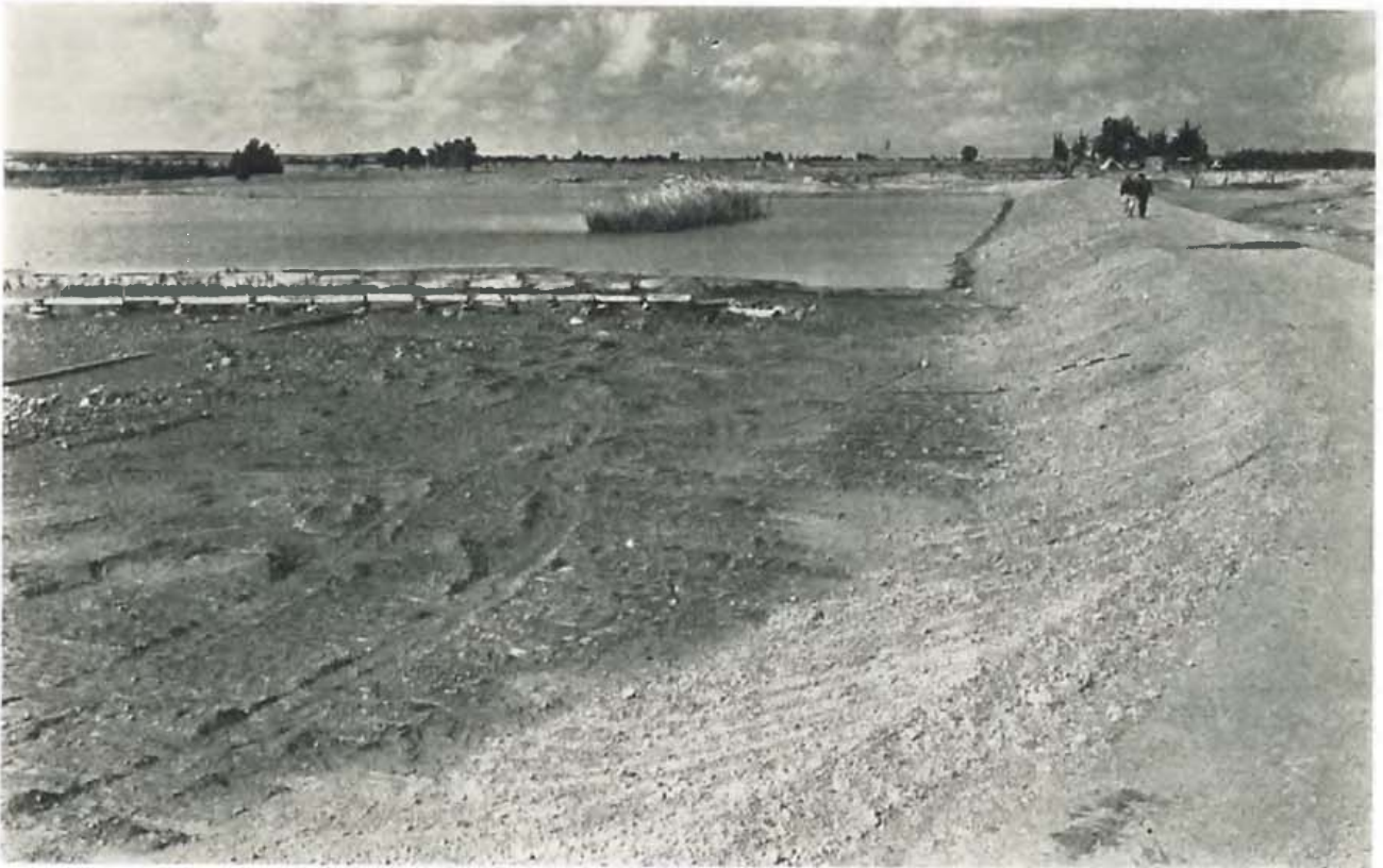
Recharge dam at Makrasyka.
