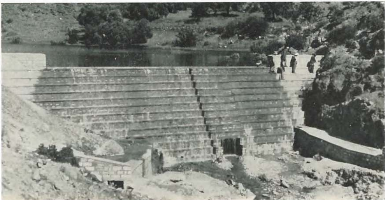
The Akrounda masonry dam.
